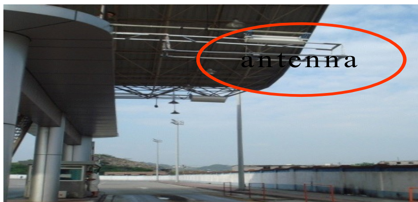
Figure 3 Antenna of RFID reader at the gate of container terminal
